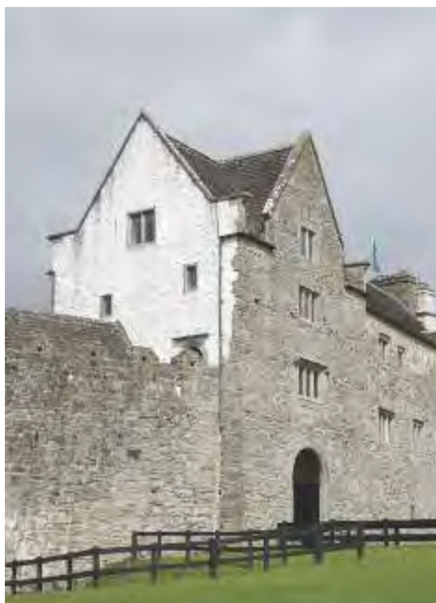
Pl. 3.8—The south and east gables of the gatehouse (Photographic Unit, NMS).
