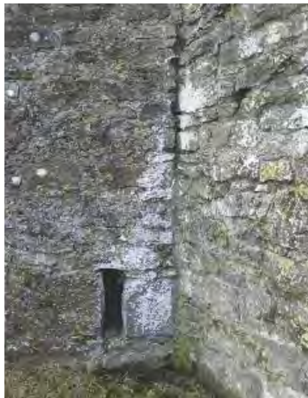
Pl. 3.17—The lack of bonding evident at the point where the north-east corner tower meets the northern bawn wall (Photographic Unit, NMS).
