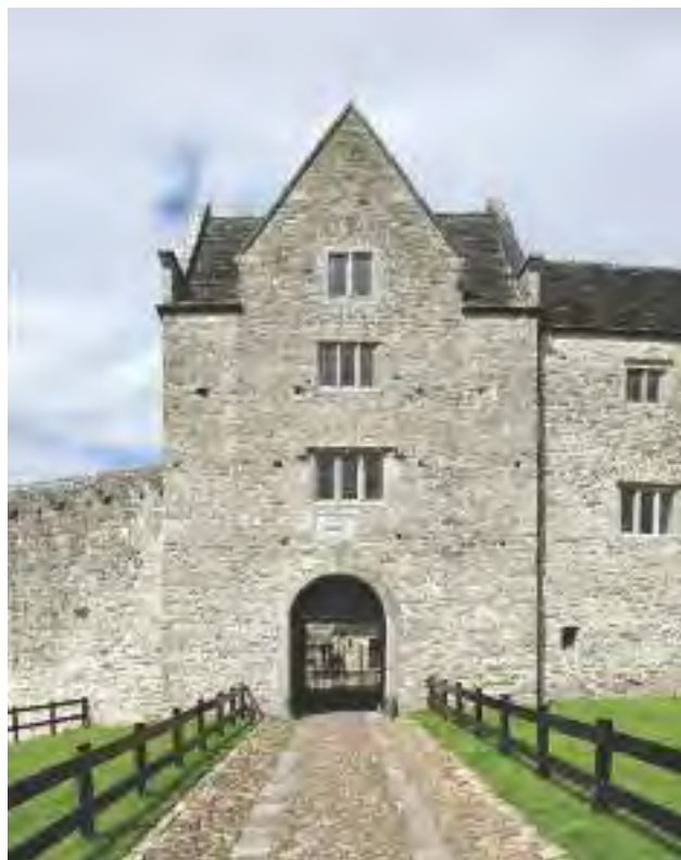
Pl. 3.3—The eastern façade of the gatehouse (Photographic Unit, NMS).
