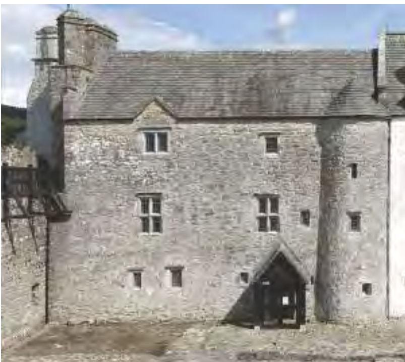
Pl. 4.23—Exterior of restored manor house from inside bawn, looking east (Photographic Unit, NMS).
