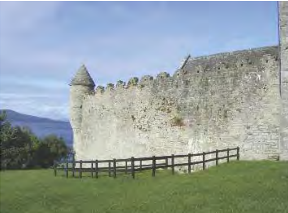
Pl. 3.29 —Exterior view of the south-eastern section of the bawn wall (C. Donnelly).
