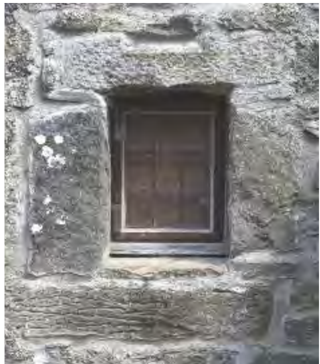
Pl. 3.13—Window in western façade of the manor house with a window-sill from an earlier building reused for the window lintel (Photographic Unit, NMS).
