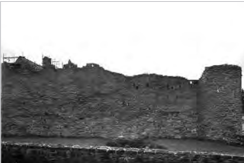
Pl. 3.22—Pre-conservation view of the northern bawn wall and north-west corner tower (Photographic Unit, NMS).
