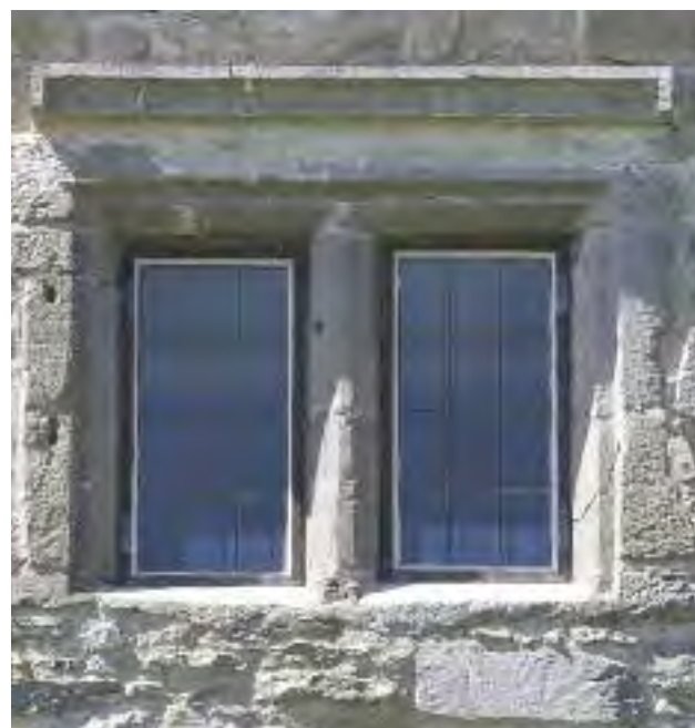
Pl. 3.11—Mullioned window in the eastern façade of the manor house, showing that the pieces have been reused from an earlier structure; note the presence of a bar-hole on the uppermost jamb stone to the left, and another set in the left side of the mullion (Photographic Unit, NMS).
