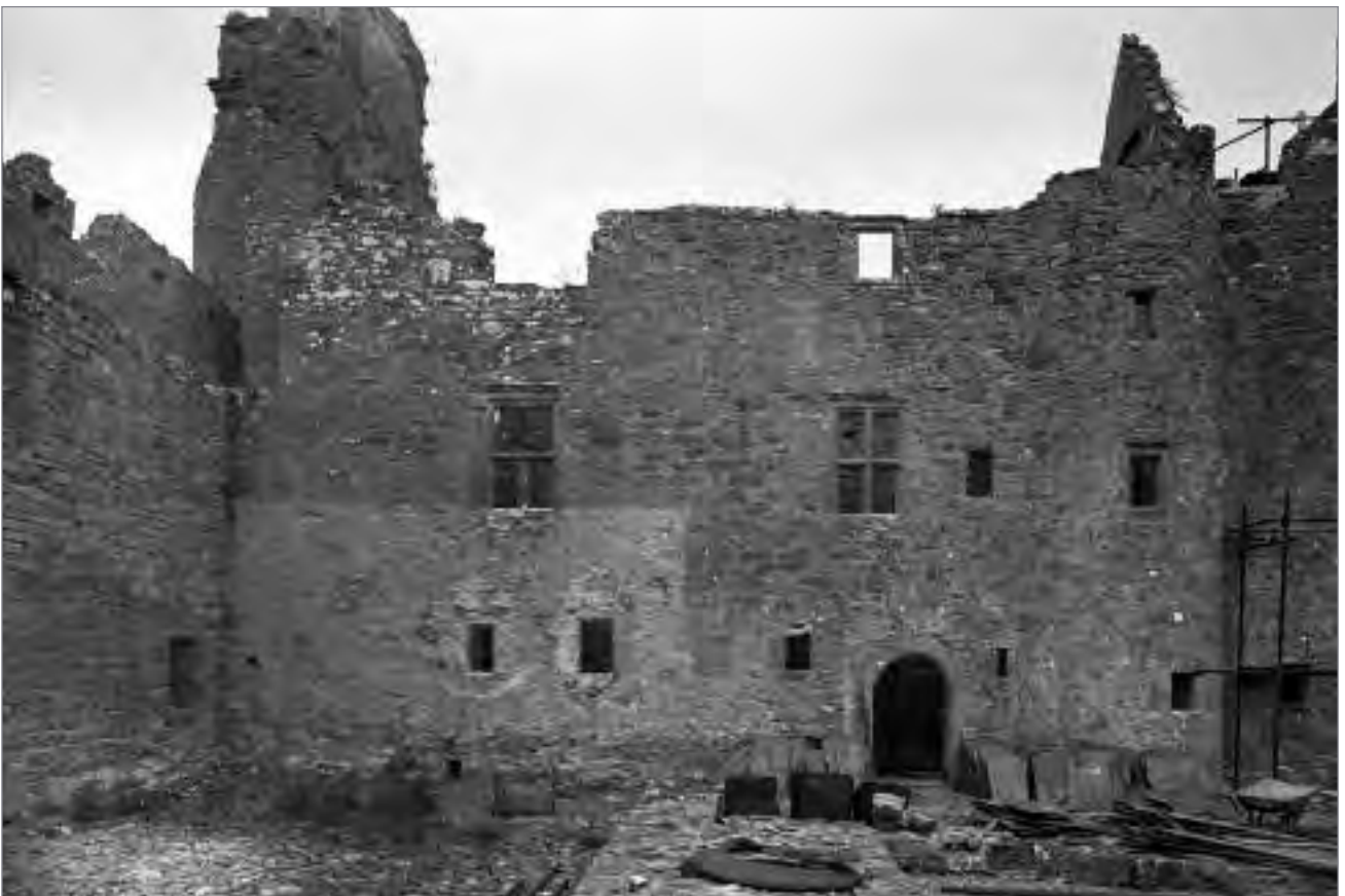
Pl. 3.16—Pre-conservation view of the interior of the bawn, showing the western façade of the manor house (Photographic Unit, NMS).
