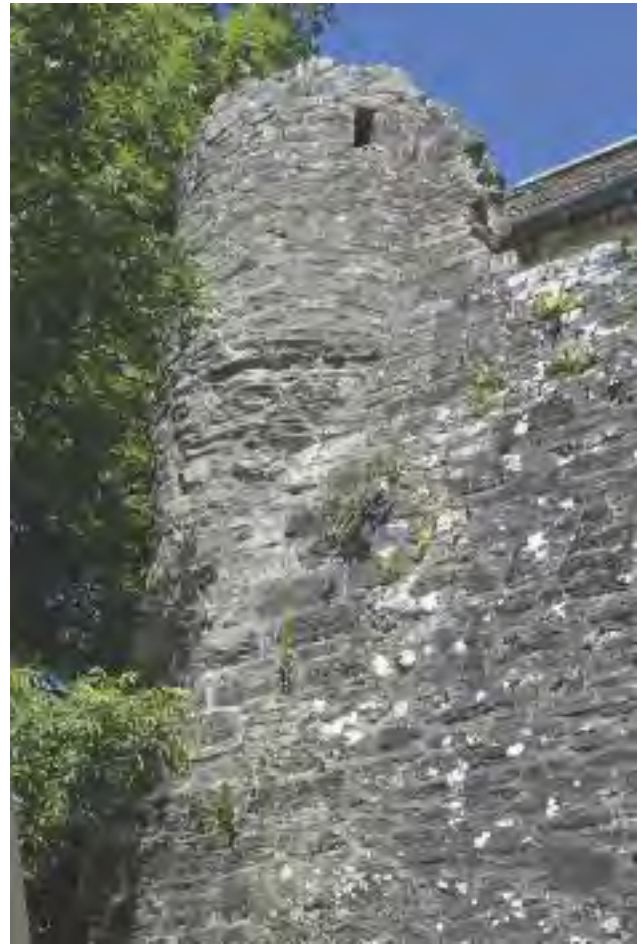
Pl. 3.32 —The south-west corner turret, roofless and unrestored (Photographic Unit, NMS).
