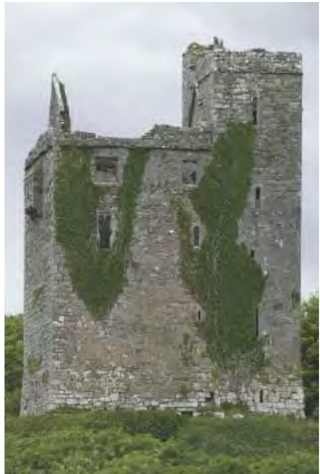
Pl. 3.26—Ballinalacken, Co. Clare, an example of a sectionally constructed tower-house (Photographic Unit, NMS).
